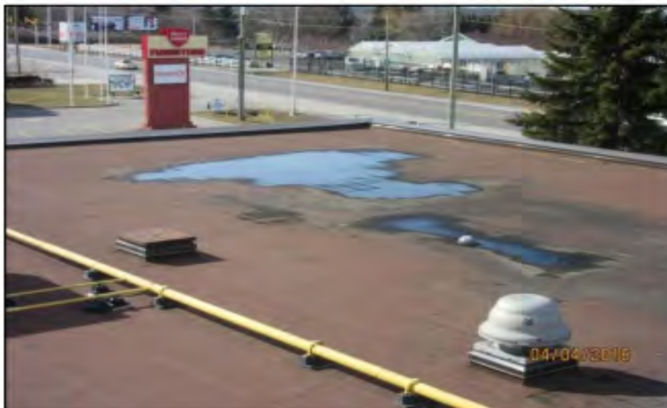
Figure 4 - 4565 Bank St (Water Pooling on Roof)
