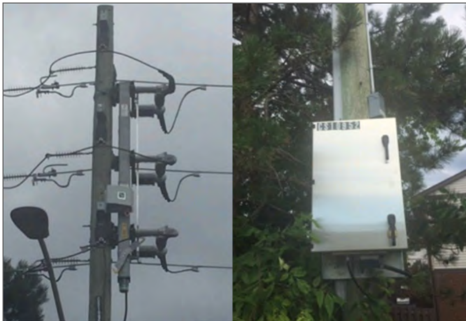
2 3 4 Figure 23 - Example of Smart FCI Device on Overhead Pole Line
