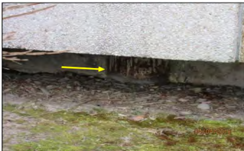
Figure 5 - 4565 Bank St (Spalling of Concrete Foundation )
