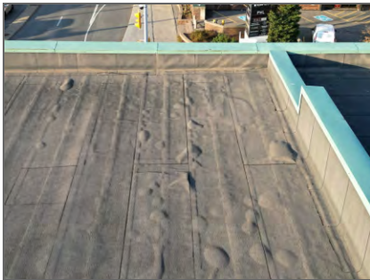
Figure 17 - Substation Roof Bubbling
