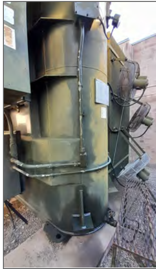
(a) Station transformer corrosion and leaks
