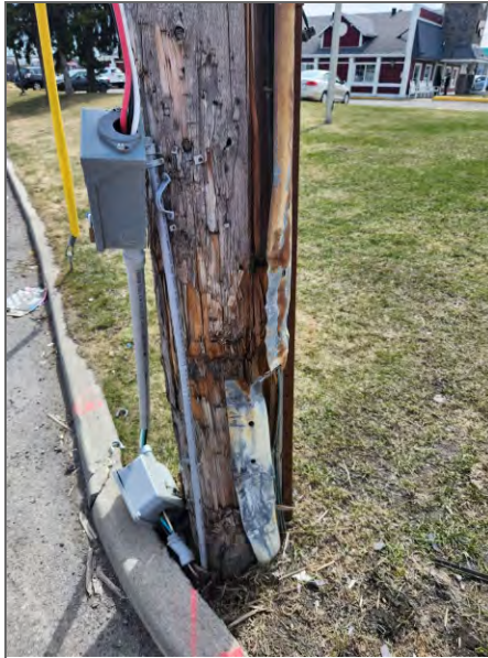
Figure 77 - Pole Damaged Due to Motor Vehicle Accident
