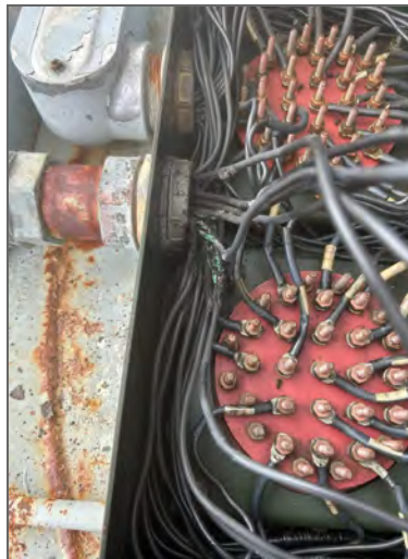
(c) Corroded connections and burnt wiring
