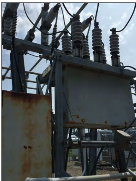
(e) Station outdoor infrastructure deterioration
