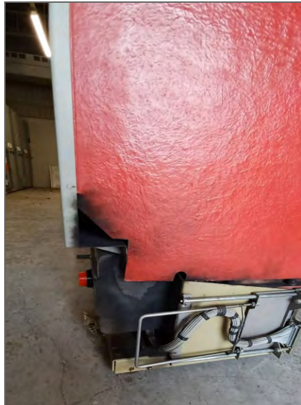
Figure 9 - FPE DST-2 Breaker Failure Event
