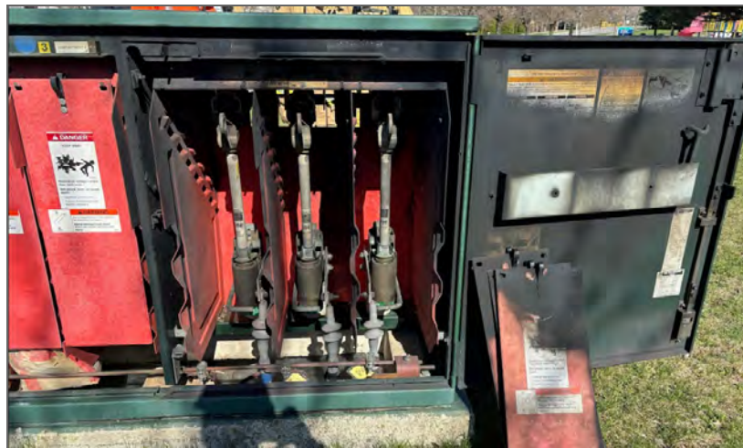
Figure 47 - UG Air Type Switchgear Failure
