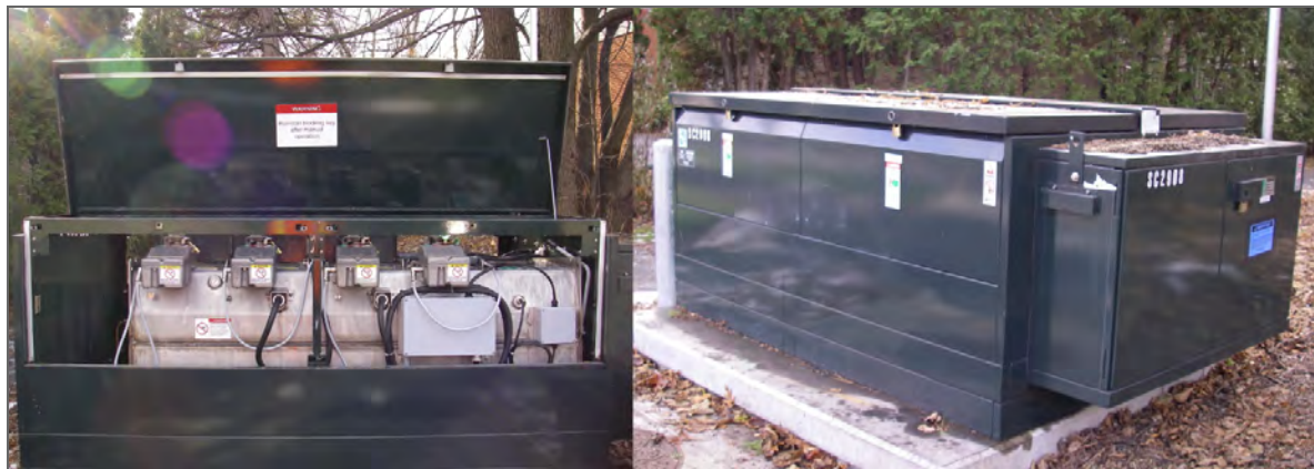
Figure 21 - Example of Automated Switchgear with Control Box
