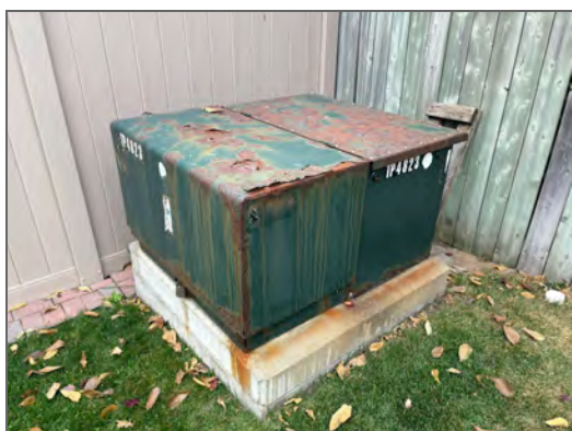
(a) Underground transformer corrosion
