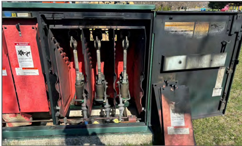
Figure 47 - UG Air Type Switchgear Failure
