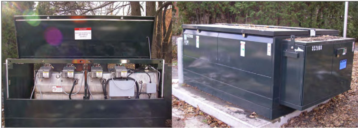
Figure 21 - Example of Automated Switchgear with Control Box
