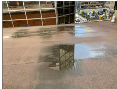
Figure 18 - Substation Roof Water Pooling
