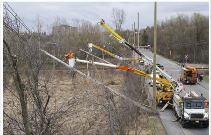
On April 28, 2011 a severe wind storm caused extensive damage to Hydro Ottawa's distribution system. More urban hydro poles were damaged than during the 1998 ice storm.
