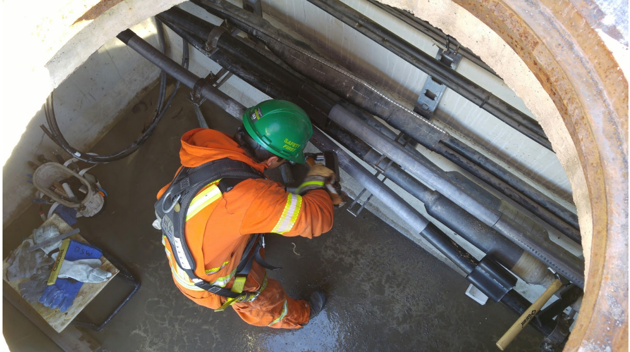
Figure 6.48 – Cable Splicing within a Cable Chamber
