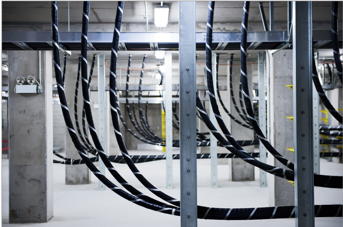
Figure 6.35 – Installation of XLPE Cable in a Station Basement
