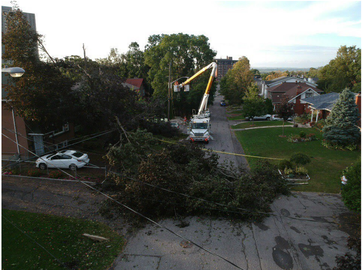
Figure 4.4 – Outage Caused by Tree Falling onto Overhead Line
