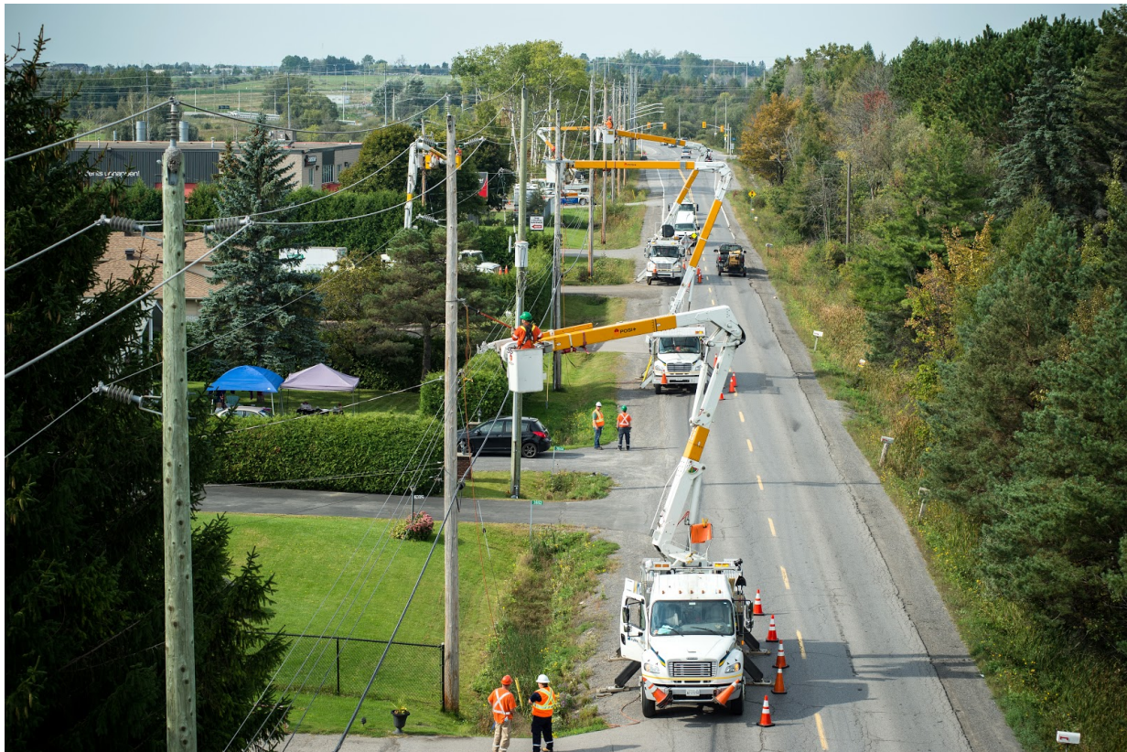
Figure 1.2 – Planned Insulator Replacement on 27.6 kV Pole Line
