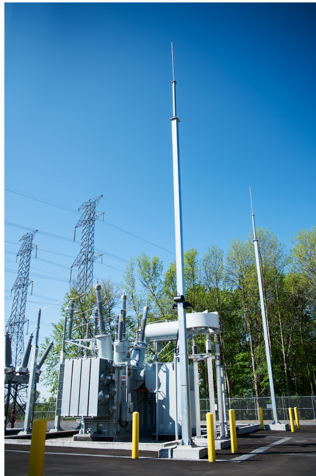
Figure 6.5 – 28 kV Station Transformer at Terry Fox MTS
