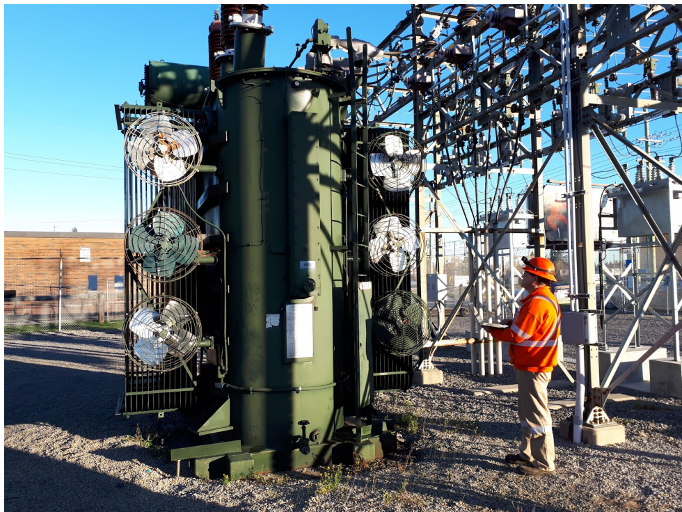
Figure 6.51 – Visual Inspection of a Station Transformer
