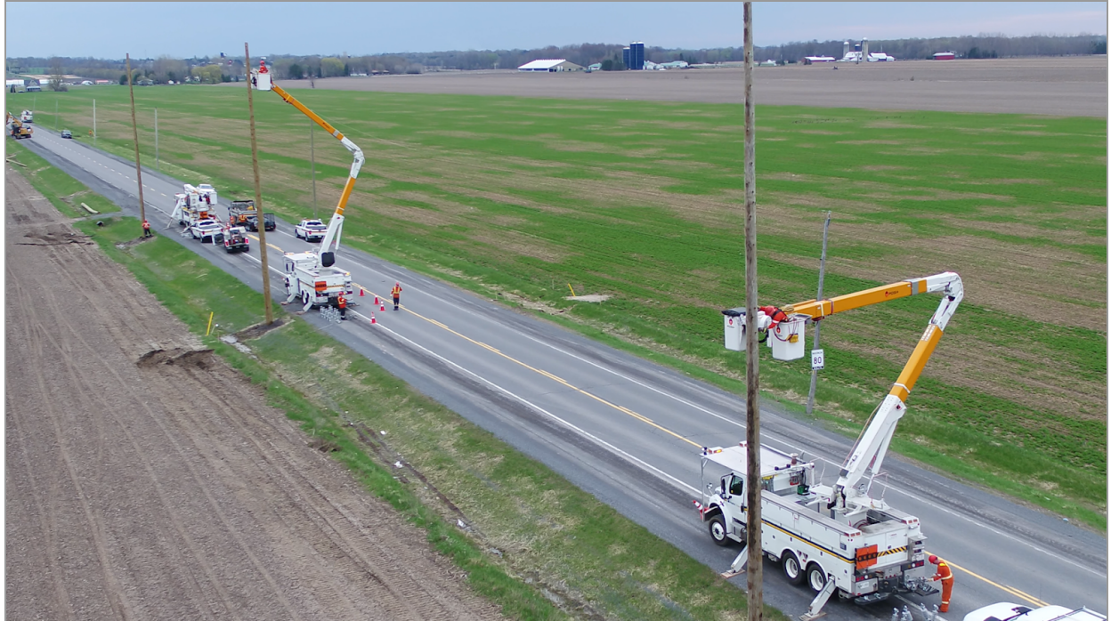
Figure 6.22 – Installation of New Pole Line
