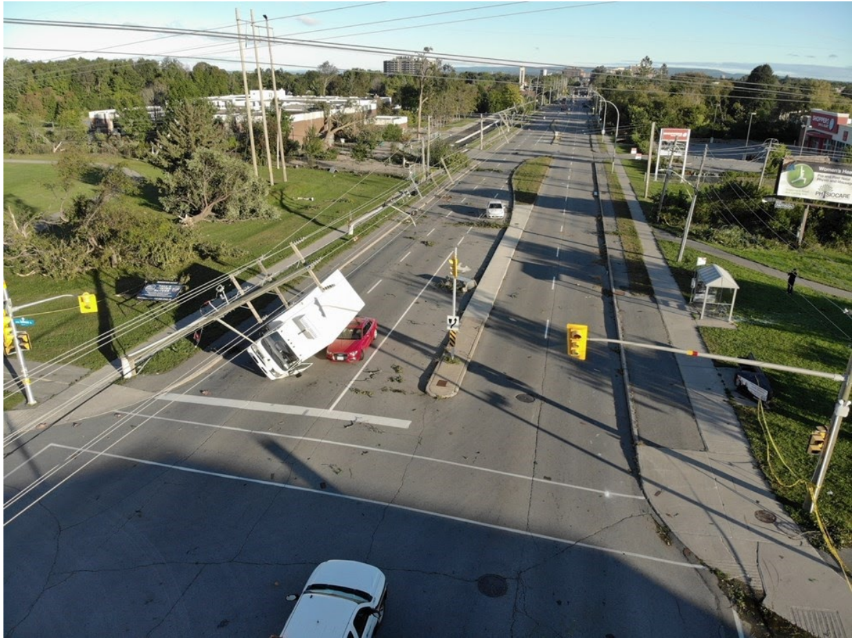
1 Figure 4.21 – Downed Pole Line Following September 2018 Tornado Event
